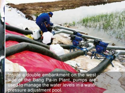
Inside a double embankment on the west side of the Bang Pa-in Plant, pumps are used to manage the water levels in a water pressure adjustment pool.
